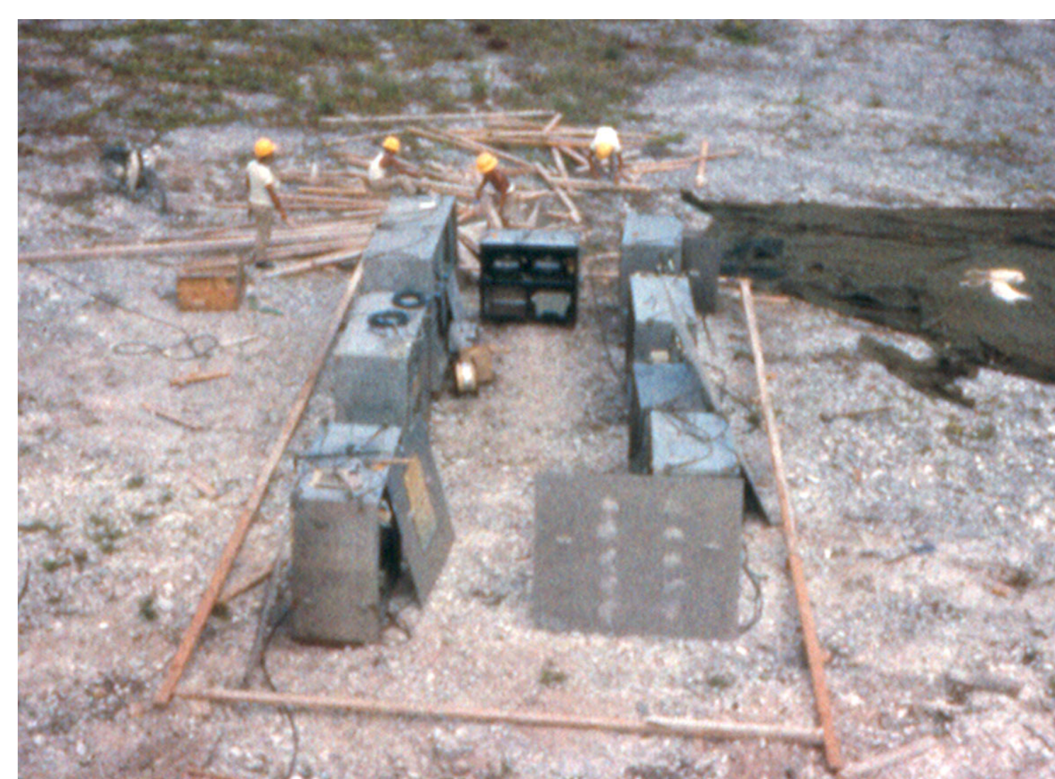
It was imperative that we send data to Maryland. This do-it-yourself TTY-(teletype)-by-radio-link equipment arrived with the tracking van. There were no instructions so no one of the tracking crew wanted to mess with it. Jerry got it working.
